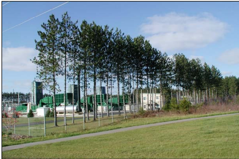
Gaylord Industrial Park's first tenant, Wolverine Power Cooperative.
